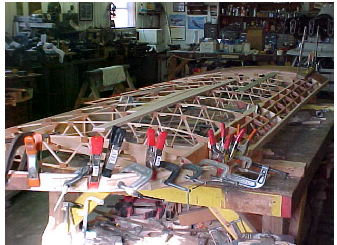
One of Tom's wings under construction at the "Rockville Waco Factory"
