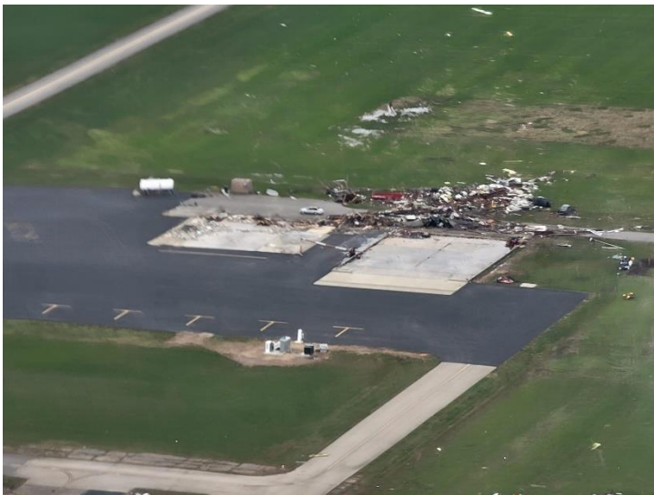
Photo showing the FBO, Maintenance and Large Hangar. Both completely removed from their foundations.
